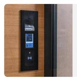
2N® IP Verso intercoms provide access to this luxury residential property. Due to its modular design, it can be configured exactly according to user requirements. For Churchill Residence, a touchscreen with Bluetooth and RFID reader was chosen, which allows users to use a mobile phone to access the building.
