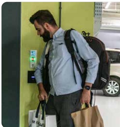
Secure access to the underground garage is provided by the 2N® IP Verso intercom in the same configuration, which is also integrated with a license plate reader (in a third-party security camera). Entrances from the garage to the corridor are then fitted with 2N Access Unit 2.0 access readers, again with Bluetooth and RFID readers.
