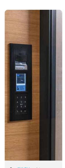
Four 2N® IP Verso intercoms were installed at the entrances. Our partner was particularly impressed by the product's modularity. In this case, the touchscreen with a treestructured directory, an RFID reader, and a keypad was also selected to provide access.
